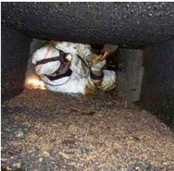
Figure 19: Checking and cleaning ductwork.
