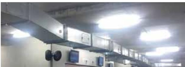
**Figure 5: Access panels every three metres in horizontal graded ductwork.**
